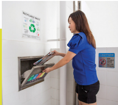
SEPARATE CHUTES FOR RECYCLABLE WASTE
