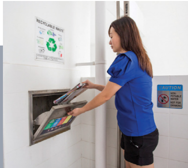
SEPARATE CHUTES FOR RECYCABLE WASTE
