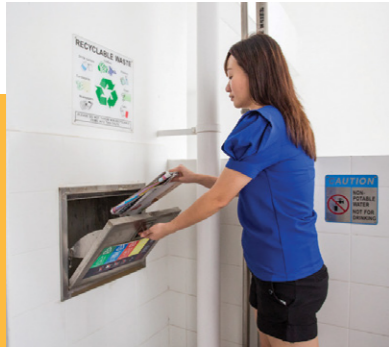
SEPARATE CHUTES FOR RECYCABLE WASTE
