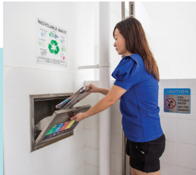
SEPARATE CHUTES FOR RECYCABLE WASTE
