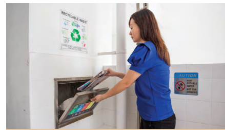
Separate chutes for recyclable waste
