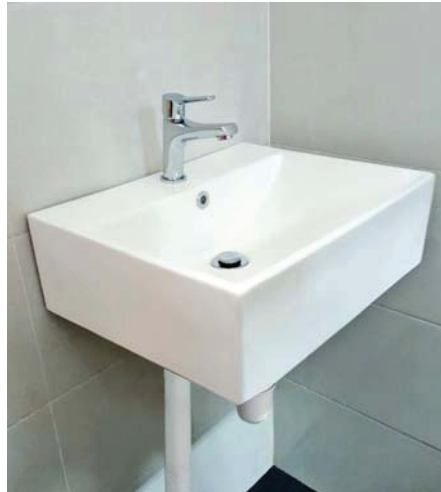
Wash basin with tap mixer
