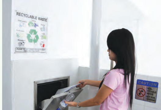
Separate chutes for recyclable waste
