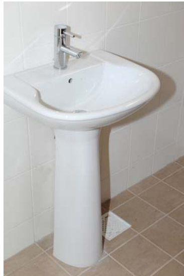
Wash basin with tap mixer
