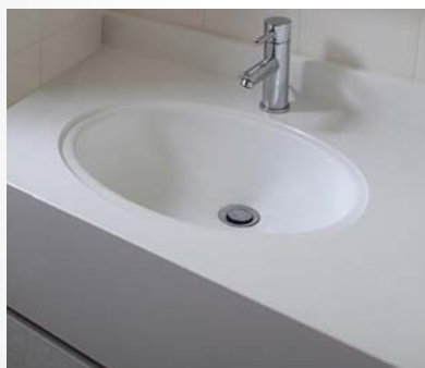
Vanity top wash basin with tap mixer in attached bathroom (applicable for 5-room and 3Gen flats)
